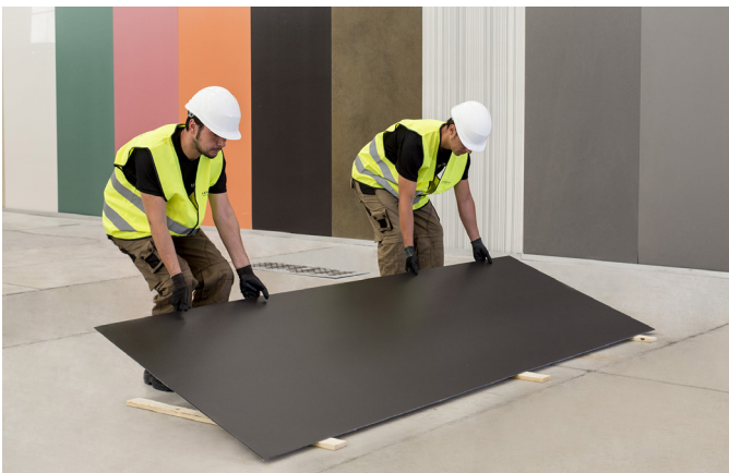
YES Spread your arms to cover as much surface area as possible and gently rest the panel on the floor.
