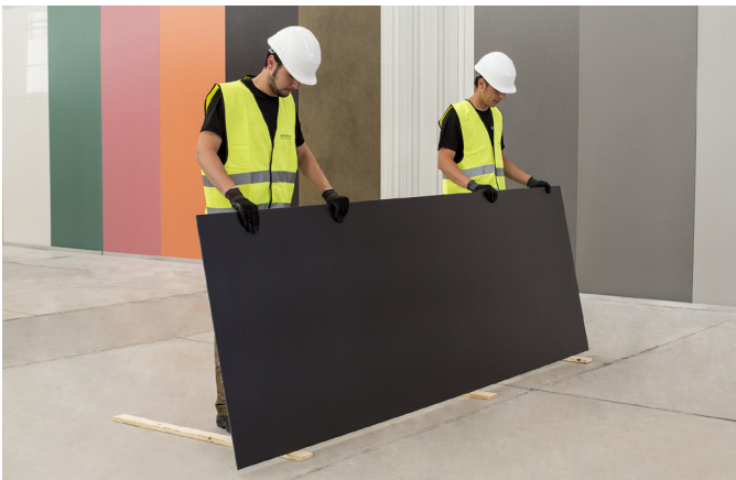
YES Position both protectors before resting the panel on the floor.
