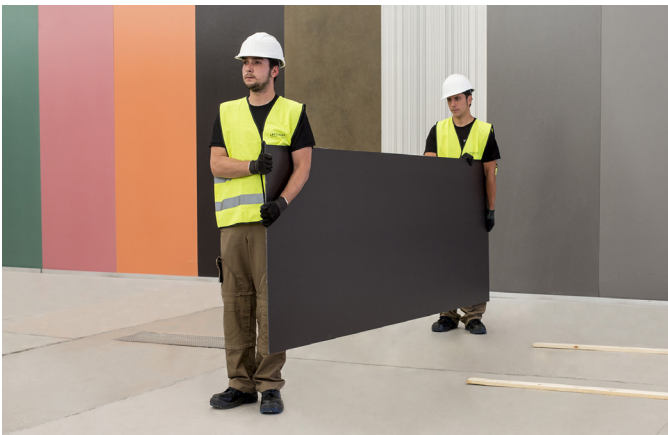
YES When the panel is vertical, lift it and keep it straight at all times.
