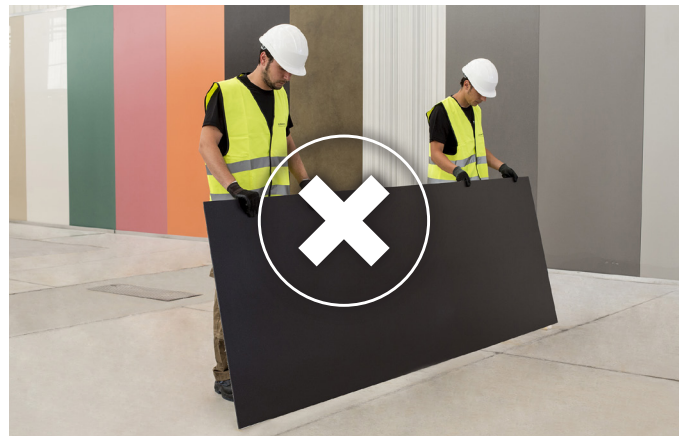
NO Do not rest the panel on the floor without the protectors.
